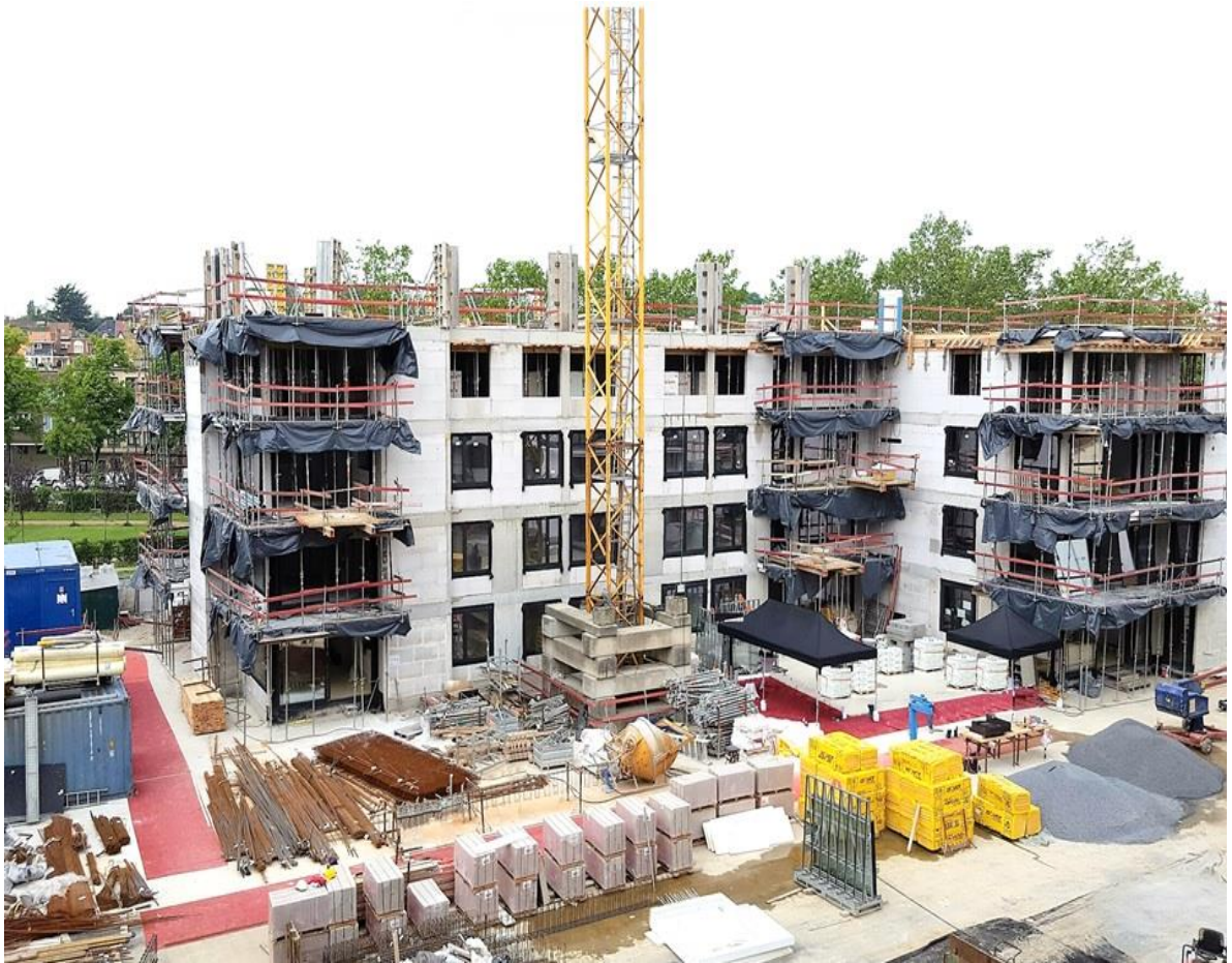
Figure 7.1.6-1 Illustration of sequenced works and 5S layout in Block 3 (block 3)
